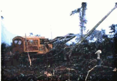
Fig. 16. Clearing operation before rubber trees are planted.
