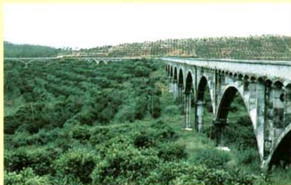
This aquaduct traversing citrus orchards near Guangzhou supplies irrigation water to both the young, recently planted orchard on the hill in the background and the productive orchard in the foreground.
