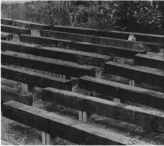
Fig. 1. Douglas-fir timbers in place on cinder blocks at the test site. Note the rows of rubber stoppers sealing the inoculation and fumigation holes.
