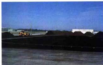
Fig. 2. Pine bark composting plant using the windrow process.
